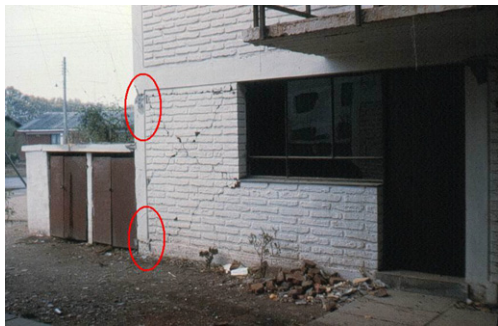
(a) Building in Melipilla city.
