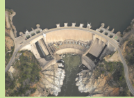
Figure A) Rapel reservoir dam
