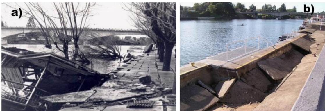
Fig. 12. Liquefaction in Muelle Schuster at Valdivia City: (a) 1960 Valdivia Earthquake (El Mercurio) and (b) 2010 Chile Earthquake (Sernageomin).
