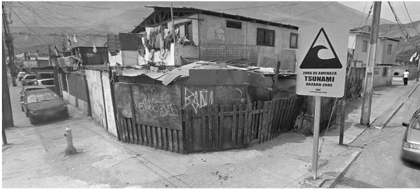
Fig. 11. Iquique: View of the Población Jorge Inostroza , located in a flooding risk area by tsunami, and on soil composed of aeolian deposits associated with a poor site response to seismic events—liquefaction susceptibility (Fig. 3). This sector corresponds to an area of high social vulnerability (Fig. 4) and it is characterized by a high density of dwellings built with precarious materials and a population in an overcrowding condition. Although this population had its origin as a campamento , today it is fully integrated into the city, forming the "Barrio Norte" of the communal regulatory plan. Photo: Google Street View, 2015.
