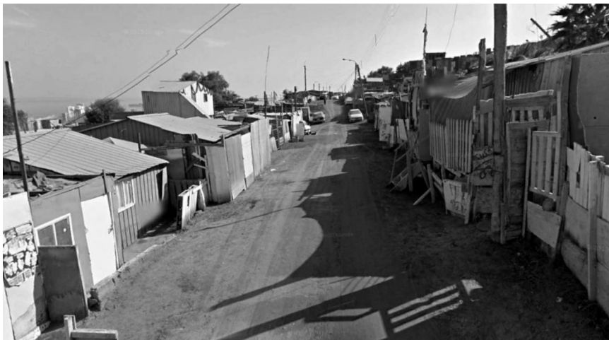
Fig. 12. Iquique: View towards the interior of Campamento Laguna Verde , located in an area that is not exposed to flooding by tsunami, but is located on the sandy mantles associated with soils with poor resistance, next to the northern side of the El Dragón dune. The dwellings have been built with precarious materials in an area with high construction density. Photo: Google Street View, 2014.
