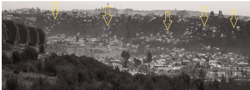
Fig. 10. Puerto Montt: Panoramic view of Campamento Ladera Lintz , located on unstable scarps with high angle gradients. According to Derch [48], the campamento is located in an area that has had at least 8 landslides. Currently, it is recommended that the construction of housing near the scarps be forbidden [39]. Arrows indicate the informal settlements' localization. Photo: Authors' personal collection, 2014.
