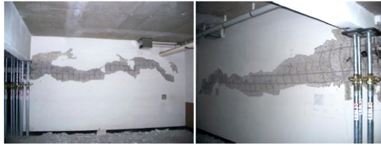
Figure 1. Damage to building walls in Chile.
