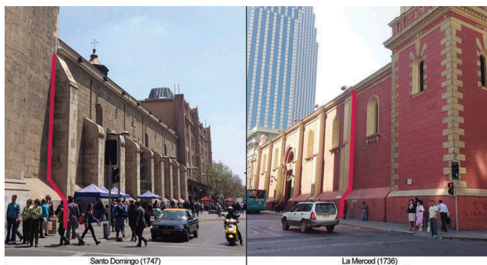
Figure 9. Buttresses and base reinforcement in the churches of Santo Domingo and La Merced.
