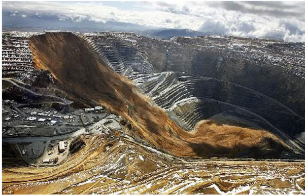
Figure 2. Landslide at Bingham Canyon copper mine in Utah, United States [3].
