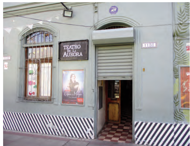
Figure 6. Barrio Italia, the continuous façade of former workers housing gives coherence and character to what was an industrial residential barrio that is now design industry, workshops and boutiques (Source: Authors)
