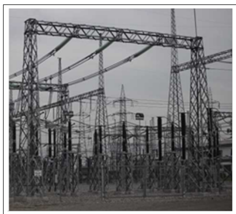
Figura 2.29: Marco Barra 220 kV [20]
