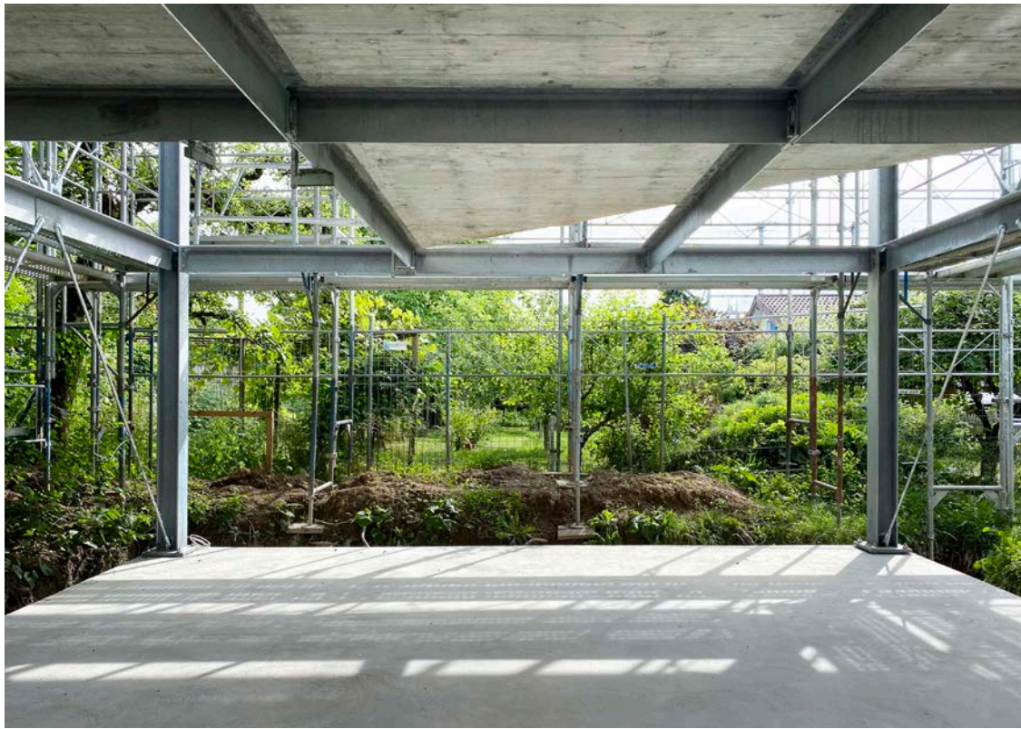
figura 3 Filter House, gentileza COMTE/MEUWLY
