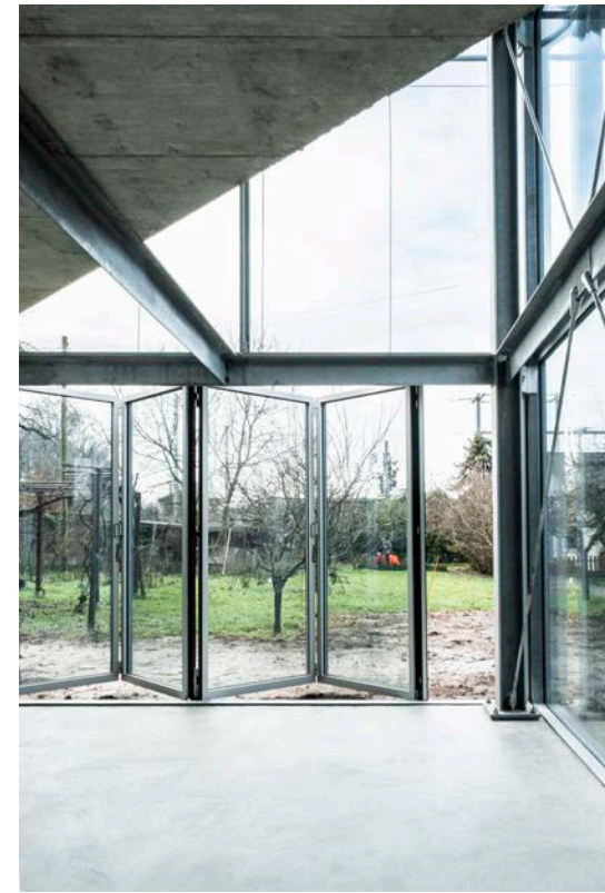
figura 4 Filter House, gentileza COMTE/MEUWLY
