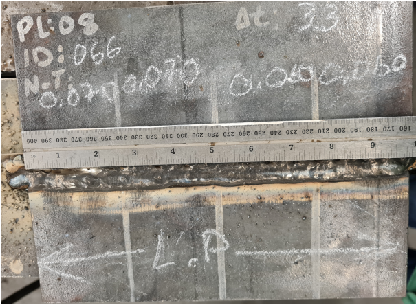
Figure 3.7: Example of a bad weld with lack of penetration taken from the eighth plate.
