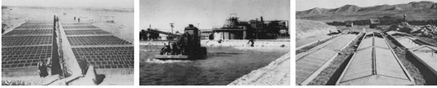
Fig. 16.1 From left to right: Solar distillation plant at Domeyko, c.1908 (Telkes, 1955); Evaporation pond at Coya, 1959 (Hirschmann, 1961); Experimental distillation plant at Quillagua, 1974 (Hirschmann, 1975)
