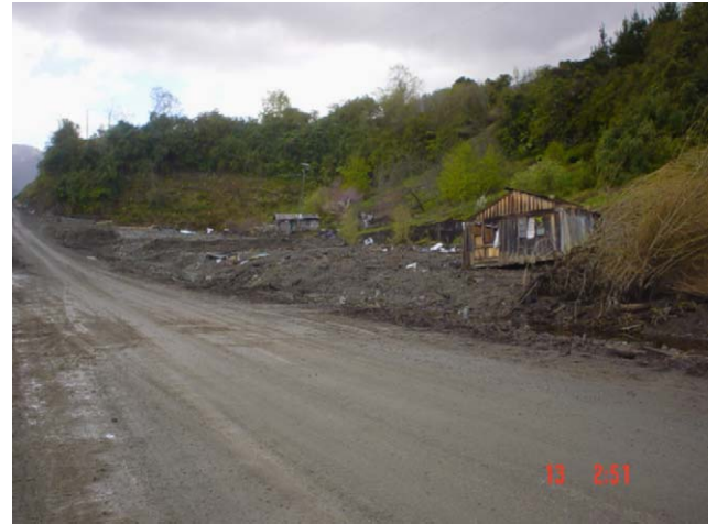
Fig. 9. View of part of the overflow of the Las Trancas Creek, Lake Ranco area, which destroyed three houses and around 500 m of road, with one fatality. The house at the right was displaced about 20 m by the flow.
