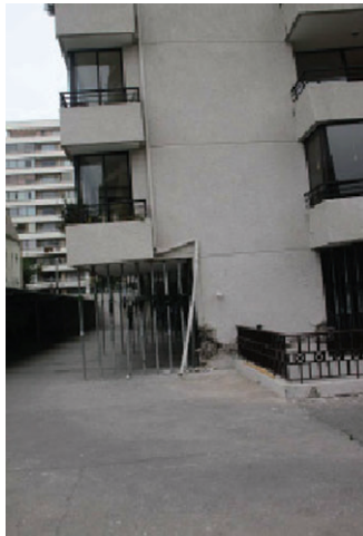
Figure 27. Toledo building: cantilevered floors and set back of shear wall at the ends of the building and corresponding interior shear walls.
