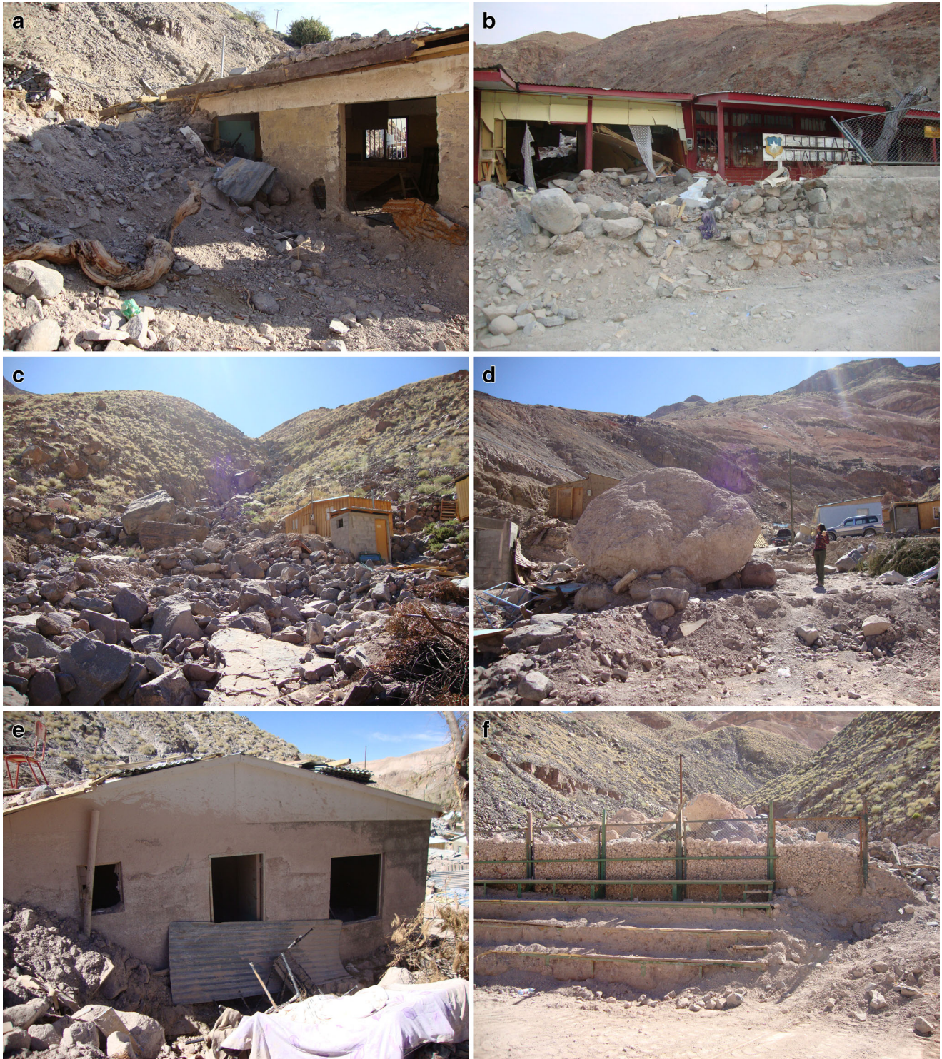
Fig. 4 Debris flows in Camiña valley. a Debris flow impact on the first upstream house in Yala Yala. Note the flow deposits on the roof; b damage by a large flow in Chapiquilta school; c Blocky flow deposit in Camiña town; d large block over 2 m in diameter in Camiña, the largest found in the urban area; e mud splash marks in the same location of the block of (d), height of about 2.5 m. The flow deposit inside the house is 0.5 thick; f sports field already cleaned and wire fence in the back that helped to retain the coarse part of a debris flow in the apex of an alluvial fan in the town of Camiña. Location on Fig. 1
