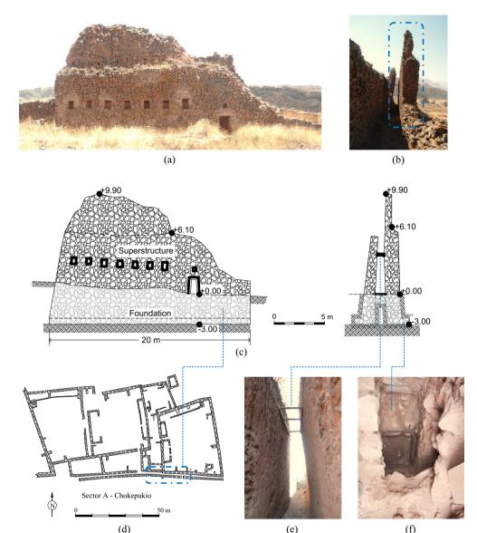
Fig. 2. General views of the studied area: (a) façade of the instrumented wall, (b) elevation of the instrumented wall, (c) front and transversal sections of the studied structure, (d) plan of the studied sector adapted from [12], (e) internal view of the two studied walls and (f) foundation detail.
