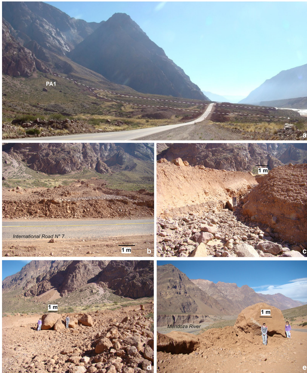
Fig. 10 Debris flows that occurred on 7 February in Picheuta area generated on alluvial fan A (Km 1173.1): a location of two tracks of PA1. b Debris flow deposit removed from the international road N°7. c Characteristics of channelized debris deposit where matrix content and boulder sizes could be observed. d , e Greatest boulders observed in the PB1 debris flow
