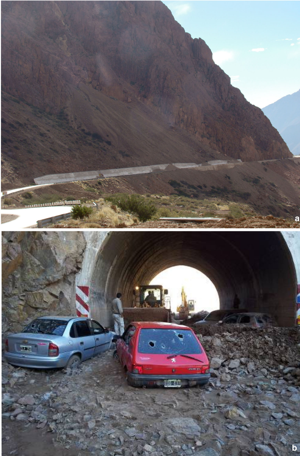
Fig. 13 Pictures of rockfalls and debris flows reported in the Cortaderas area: a rockfall generated from talus cones passing over a contention wall along 1.5 km of international road, and b rockfall in tunnel 13 burying four cars (Km 1,178)
