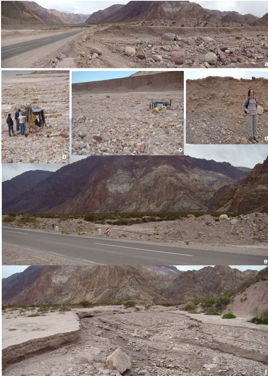
Fig. 12 Pictures of the channelized debris flows in different parts of the Quebrada Seca alluvial cone system: a hyper-concentrated flow QS1 (Km 1,171) that severely impacted on international road. b Detail of bulldozer buried by the QS1 its path into the Mendoza River. c Both bulldozers buried by the flow. d Debris material with abundant matrix content (50 %). e Debris flow channelized into another channel invading the road due to culvert obstruction. f Minor debris flow coming from the northernmost channel
