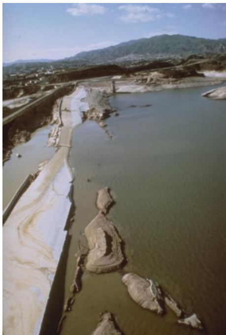
Fig. 2-7 Presa San Fernando en 1971 (NOAA National Geophysical Data Center).
