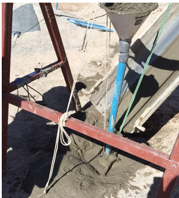
Figure 3.6: Grouting process
