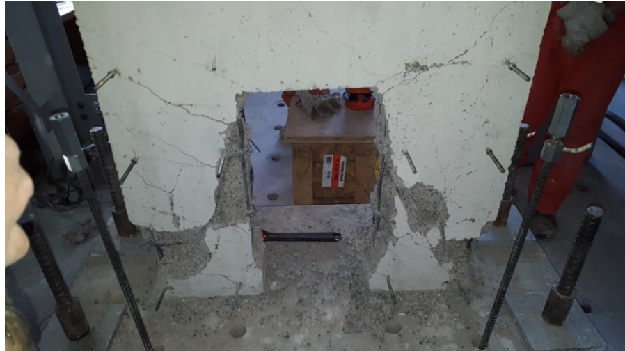
Figura 0.31: Falla cara LVDT MR3.
