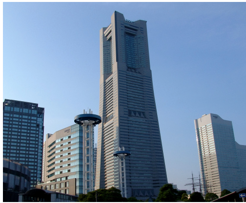
Figura 1.14: Yokohama Landmark Tower
