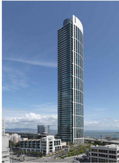
Figura 1.10: One Rincon Hill Tower
