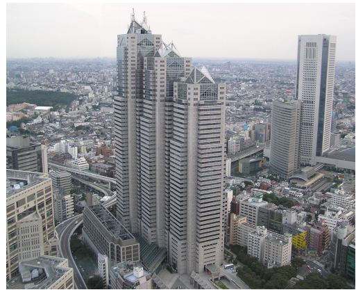
Figura 1.15: Shinjuku Park Tower
