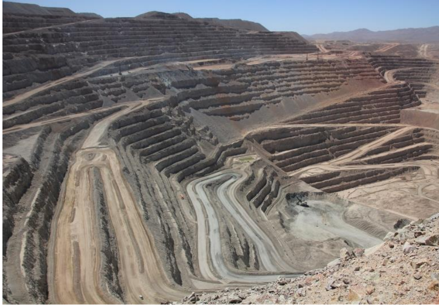
Figure 1.1: An example of open pit. Escondida, operated by BHP Billiton. Source: author.
