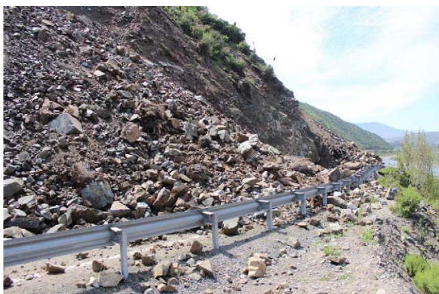
Figure 13. Traffic discontinued on Route D-75 as a result of rockfalls. Estimated volume > 200 m 3 (31.5855°S, 71.4674°W).
