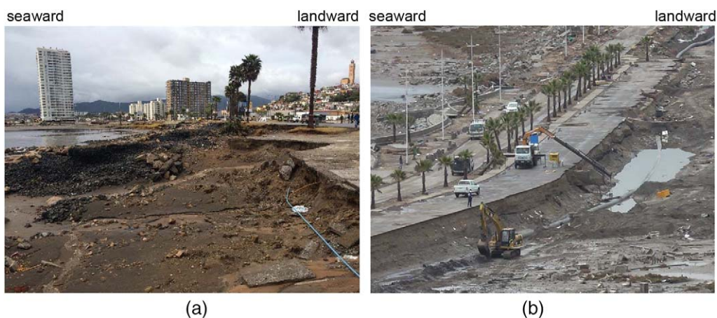
Figure 15. (a) Sand and rock fills in Coquimbo's shoreline washed away by tsunami waves (29.956°S, 71.336°W), and (b) tsunami erosion and scour along Avenida Costanera, Coquimbo (29.961°S, 71.328°W).
