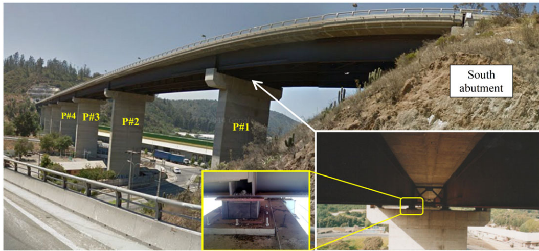
FIGURE 1 Photo of the Marga-Marga Bridge in Viña del Mar, Chile [Colour figure can be viewed at wileyonlinelibrary.com]
