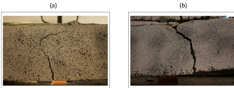
Fig. 9. Failure mode – (a) specimen A1 and (b) specimen A2.
