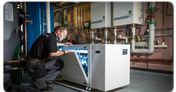
PCK80 Generator Kit integrated within a (mCHP) Micro Cogeneration System
