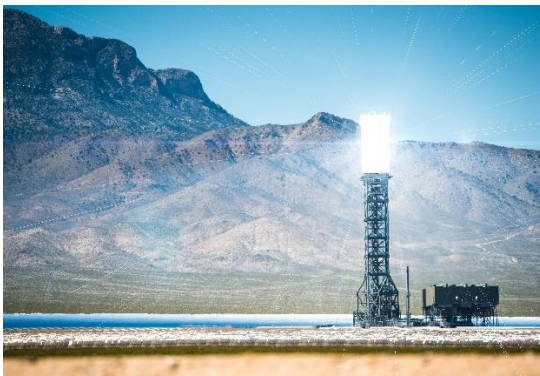
Figura 18: Receptor solar externo [14]
