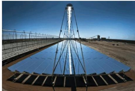
**Figura 3:** Colector lineal Fresnel. Fuente: US Energy Department.
