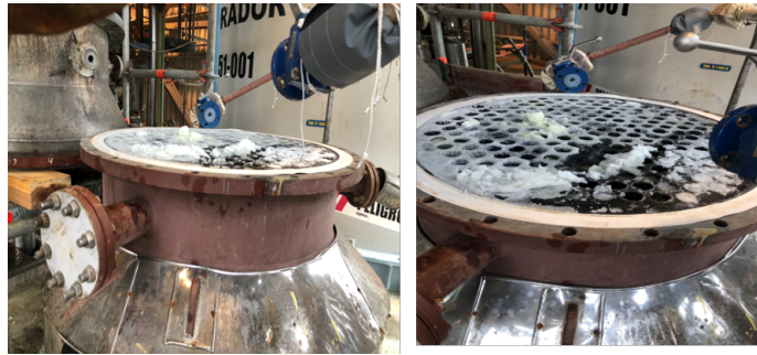
Figure 5.1: Sulphate inlays in the interior of the reboiler tubes.
