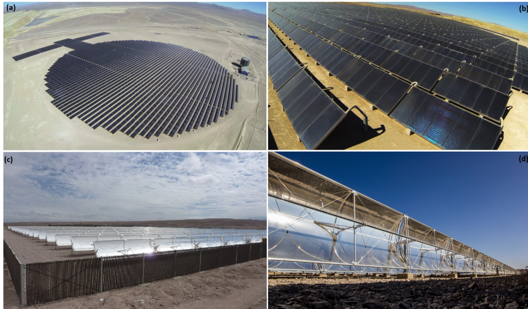
Fig. 8. Solar thermal plants for the mining industry in Chile. Fig. 6a and b show Pampa Elvira Solar. Fig. 6c and d show El Tesoro (Ellaima, 2015; Futuro Renewable, 2014; Interempresas, 2013).
