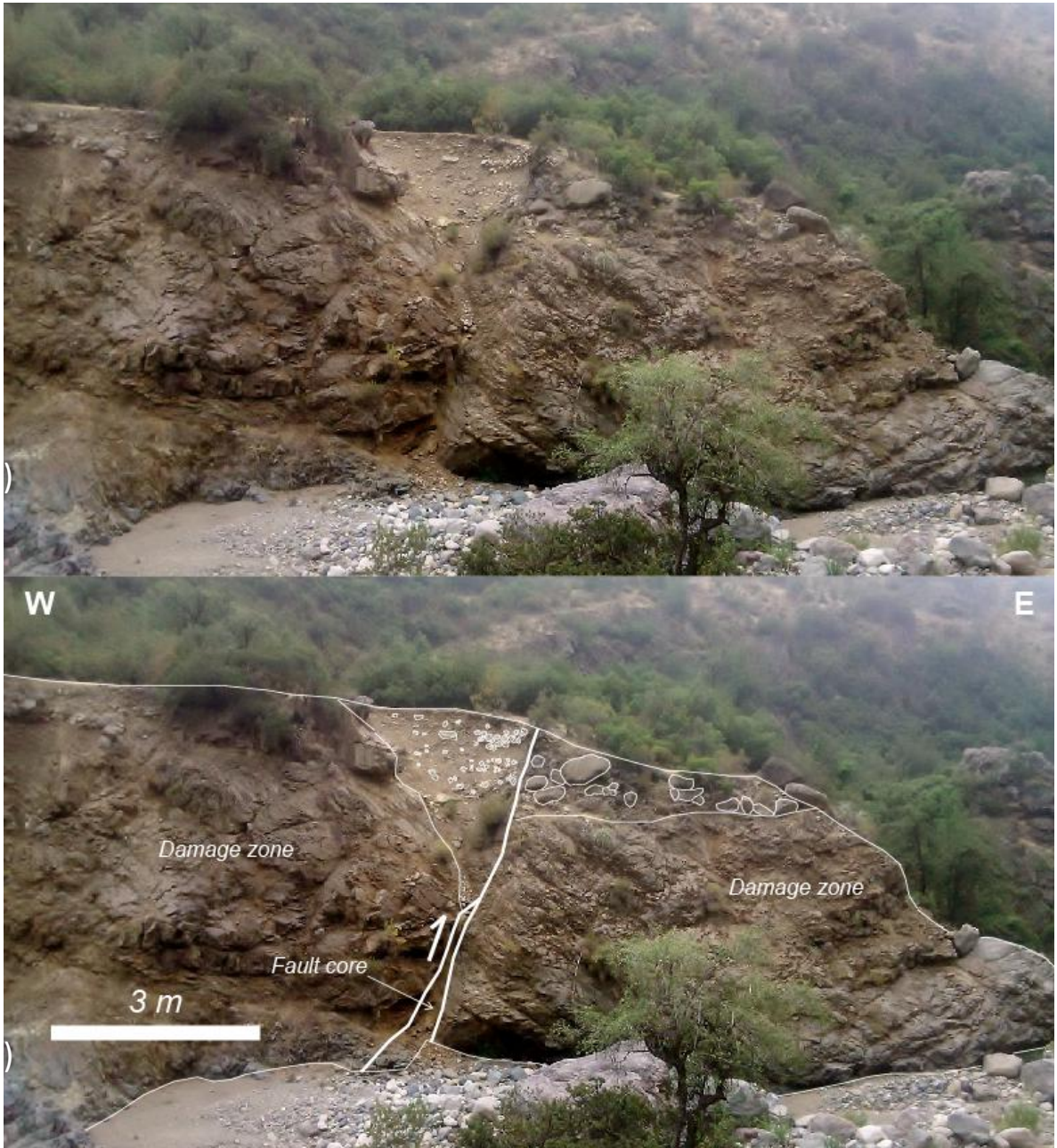
Figure 4.7 FC3 configuration indicating fault core damage zone and Quaternary deposits.
