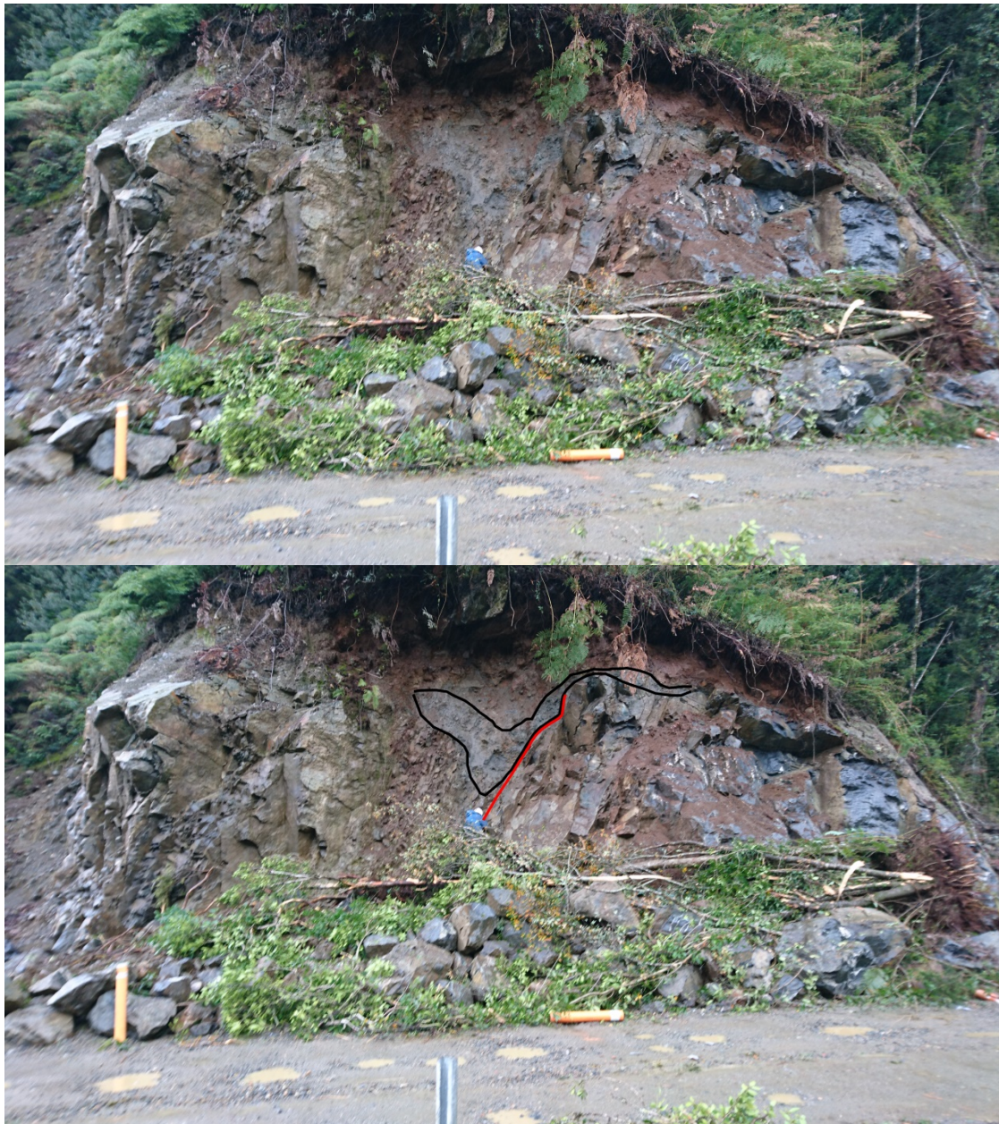
Figure 3.8. Field photograph of the Queulat fault looking south. The photo shows a grey silt layer (black lines) falling into the fault zone. The red line corresponds to the Queulat Fault plane. Note person below the fault plane for scale.
