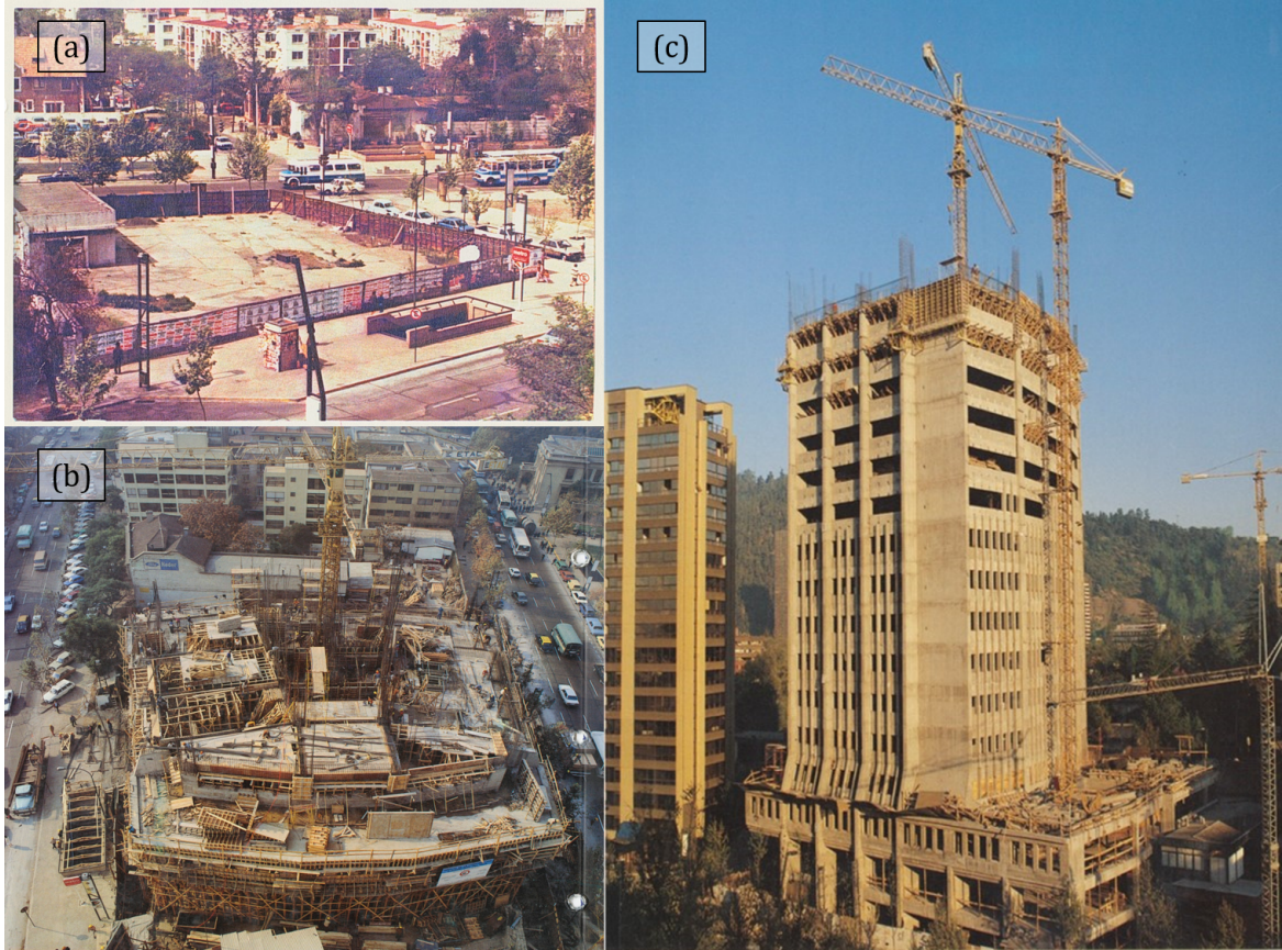
Figure 3.2: The Chilean Chamber of Construction Building during its construction (1987).
