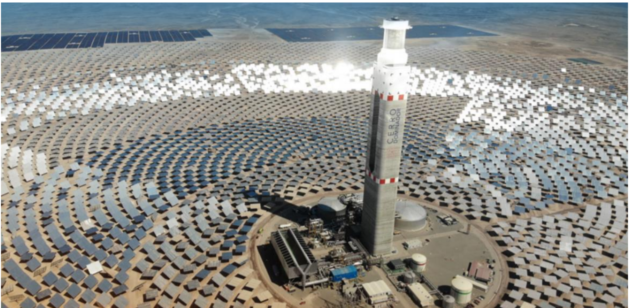
Figure 23: CSP-PV hybrid power plant Cerro Dominador, Maria Elena/Chile [41]
