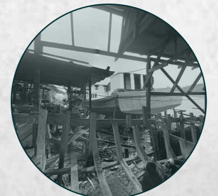
Vista interior astillero
