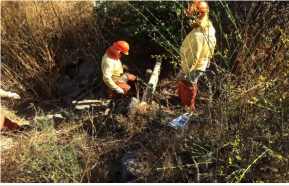
Figure 12. Bucking and Installing Palisades. Los Coipos Estate.
