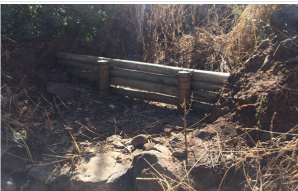
Figure 13. Palisade Completed. Los Coipos Estate.
