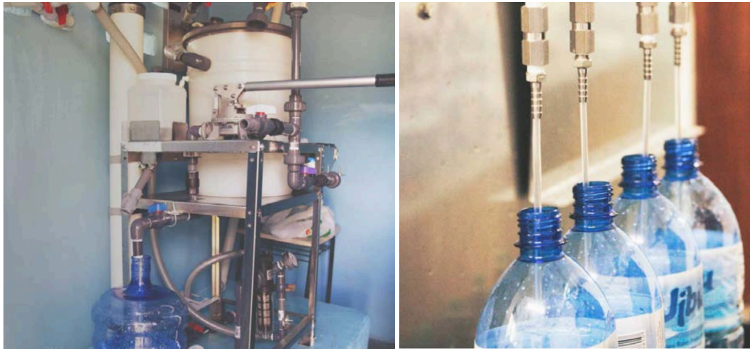
Figure 2.6 Water treatment system and filling bottles [49]
