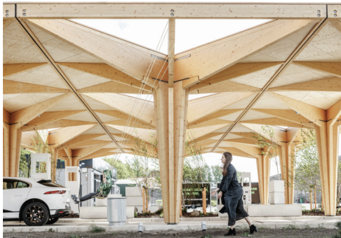
Fig 58 y 59: Fast Charging Station for Electric Vehicles / COBE Fuente: ArchDaily
