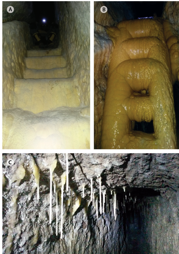
FIG. 13. A y B. Calcium carbonate covering carved steps and iron ladder in El Carmen socavón . C. Stalactites in El Sauque socavón .
