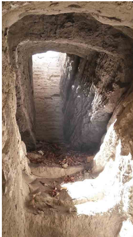
FIG. 5A. Typical shaft well ( lumbera ) in the Pica area.
