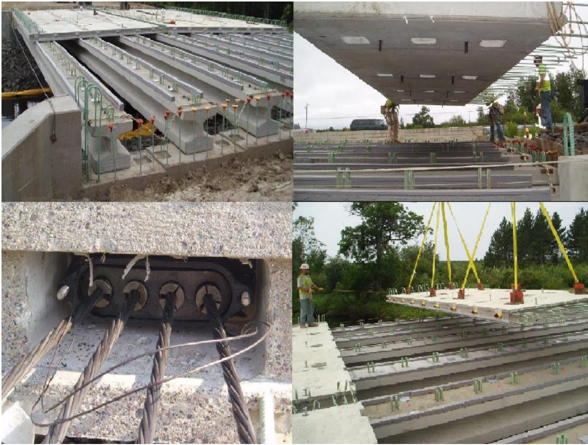
Figura 6: Puente Masatuses ABC. Fuente: Masatuses Department of Transportation.
