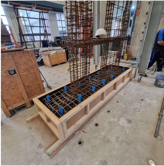
(a) Encofrado pedestal.
