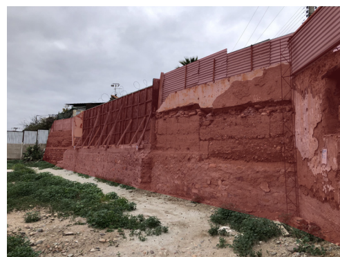
Muro interior calle Cantournet.
