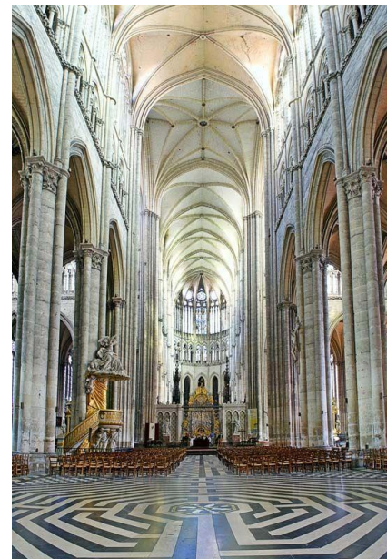
(b) Interior de nave central
