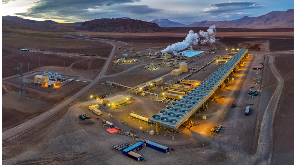
Figure 1.1: Panoramic view of Cerro pabellón geothermal power plant in Chile. Figure from Enel.cl
