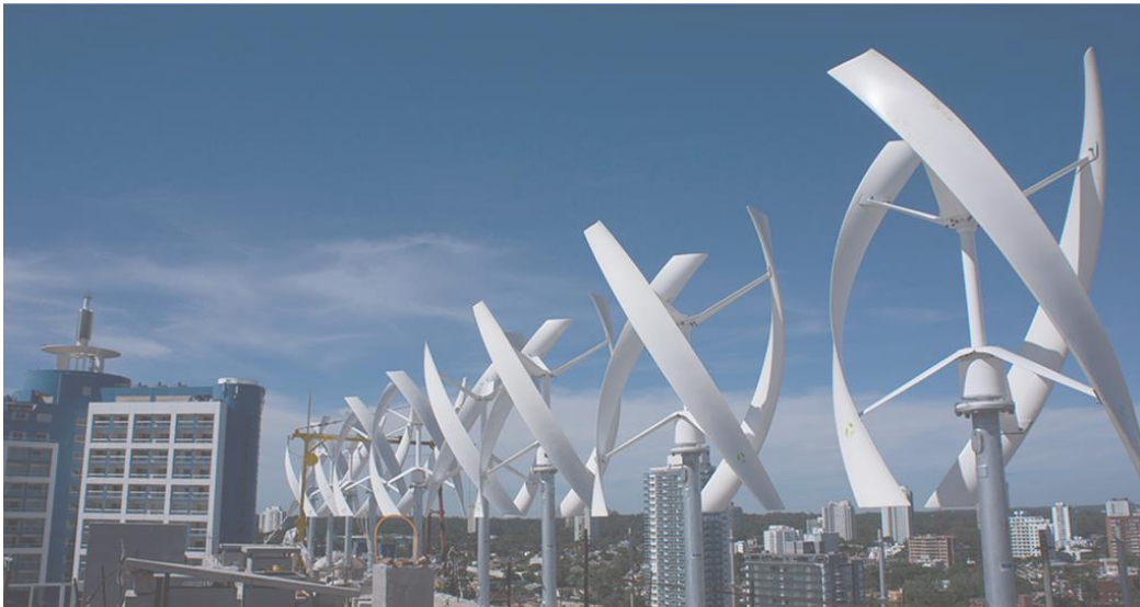
Figura 03: Azotea eólica del Edificio Alexander, Uruguay. Extraído de: Alexander Building - Wind energy generated by windmills | ... | Flickr
