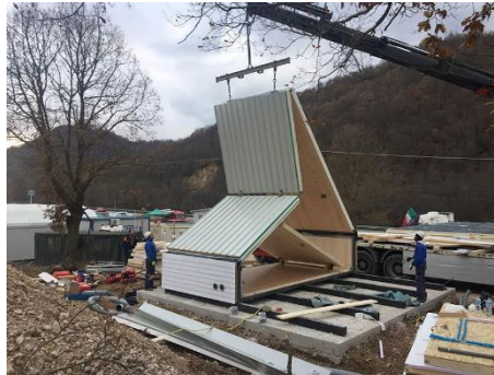
Figura 8: Nota. Adaptado de Italian Architect Designs Folding House That Can Be Built in 6 Hours por Ciclovivo, 2017, Arch Daily ( https://www.archdaily.com/885915/italian-architect-designs-folding-house-that-can-be-built-in-6-hours )
