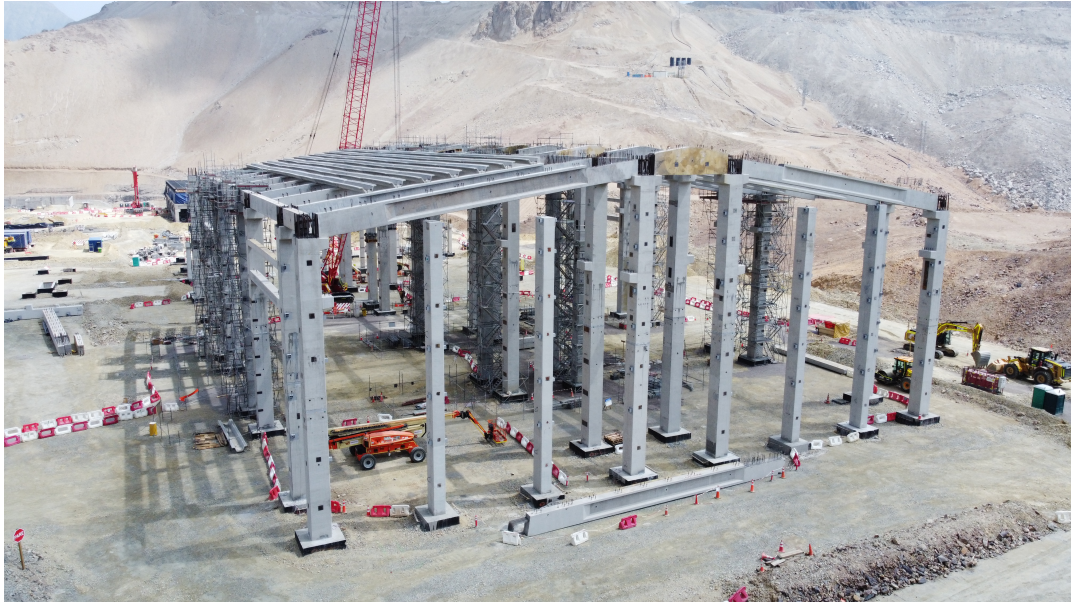
Figura 8.6: Foto 4 truck shop
