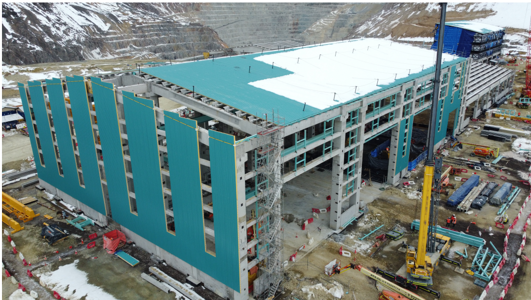
Figura 8.3: Foto 1 truck shop
