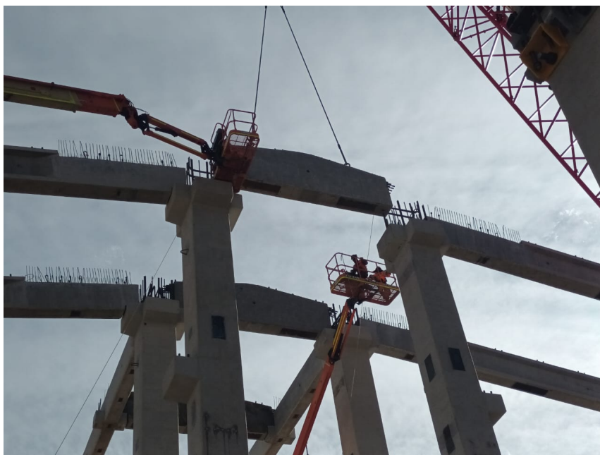
Figura 8.13: Foto 11 truck shop
