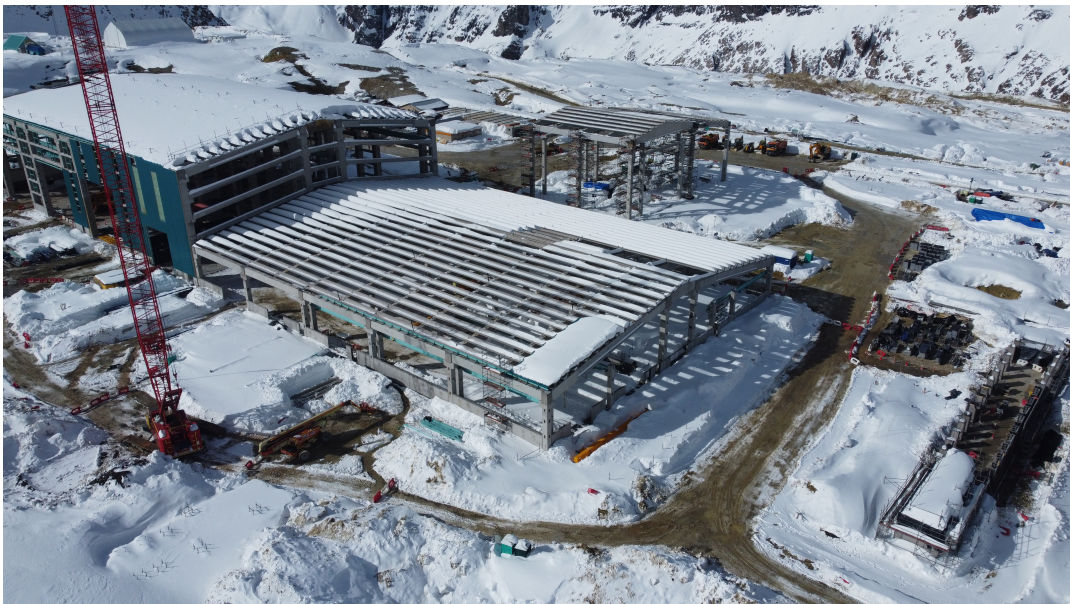
Figura 8.5: Foto 3 truck shop
