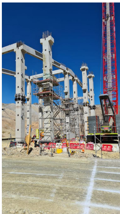
Figura 8.12: Foto 10 truck shop
