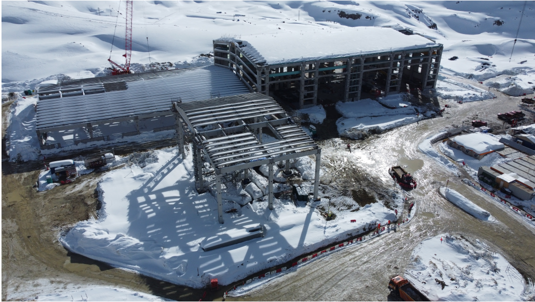
Figura 8.4: Foto 2 truck shop
