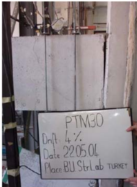
PCI Journal "Behavior of Unbonded Post-Tensioned Precast Concrete Connections with Different Percentages of Mild Steel Reinforcement" (ref. 15)
