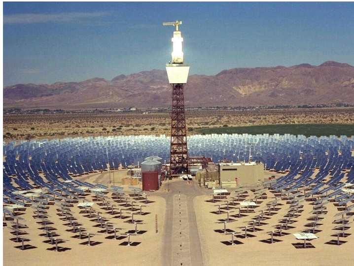
Figura 2.2: Solar Two, USA
