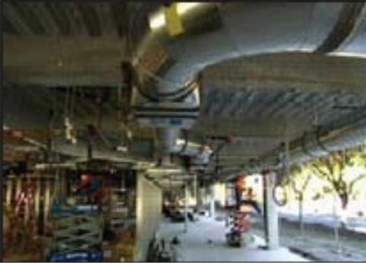
A photograph of the actual installed HVAC ducts in a building, showing that the physical installation matches the 3D BIM model. |
